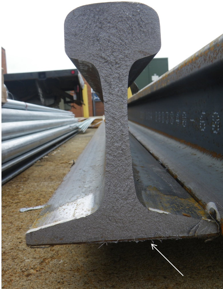
Figure 39. Resonant Fatigue Fracture Surface of Unprotected, Corroded Rail (Sample RS3) Arrow Shows Crack Zone
