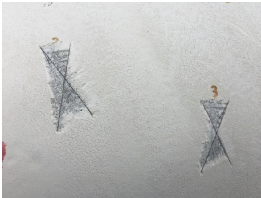
Figure 4 – Cross-cut adhesion of EonCoat – June 2018 after 4 months of being insulated and in service.
