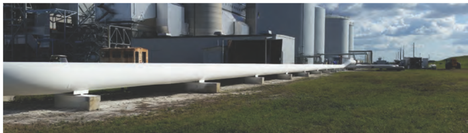
After coating with EonCoat, the substrate is covered by a ceramic shell that resists corrosion, fire, water, abrasion and caustic elements, as well as over-hot temperatures.
