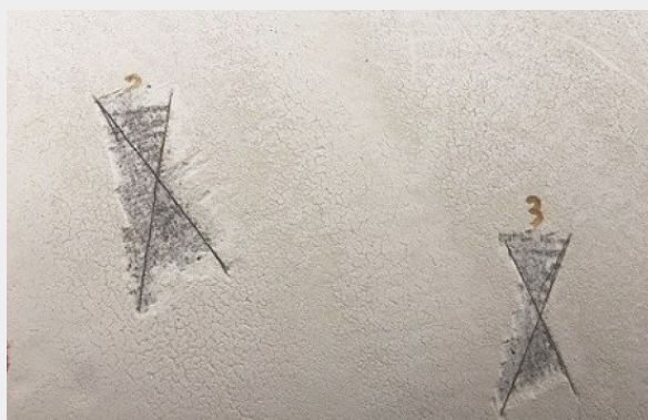
A cross-cut adhesion into the coating was examined four months after the pipe had been placed back into service. Photo courtesy of EUROCORR 2018.
