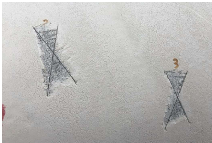
A cross-cut adhesion into the coating was examined four months after the pipe had been placed back into service. Photo courtesy of EUROCORR 2018.
