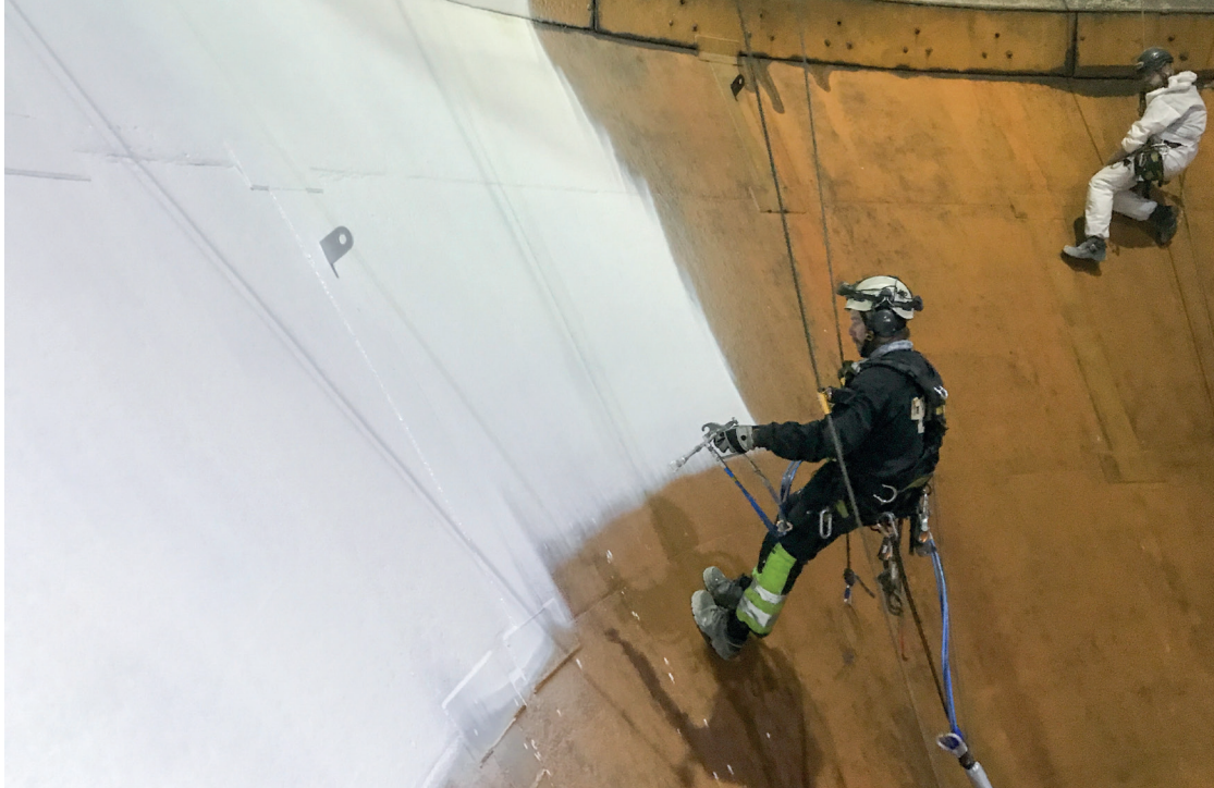
The EonCoat anti-corrosion coating was applied to the lower section of the steel hopper in a single coat at a thickness of 800 microns over an eight hour shift
