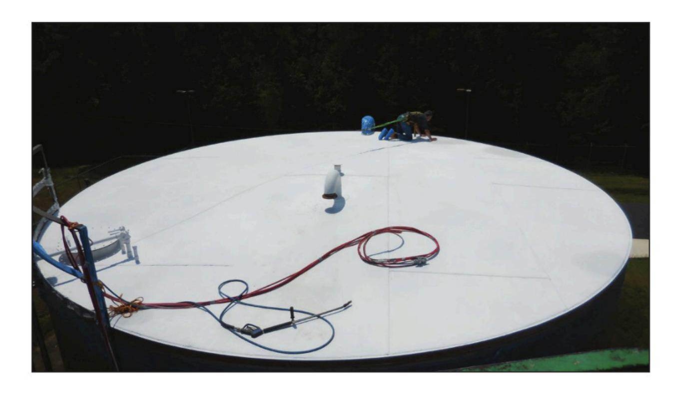
prepared, if gouged, moisture and oxygen will migrate under the coating's film from all sides of the gouge.
