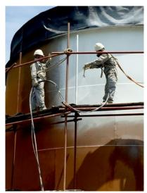
CUI, which involves the corrosion of vessels or piping beneath insulation due to water penetration, is insidious because it can remain undetected until the insulation is removed for inspection or leaks occur. Water penetration can result from many causes including monsoons, rain, flooding, wash downs, and sprinkler systems, as well as exposure to steam, humidity, or frequent condensation and evaporation of atmospheric moisture.
