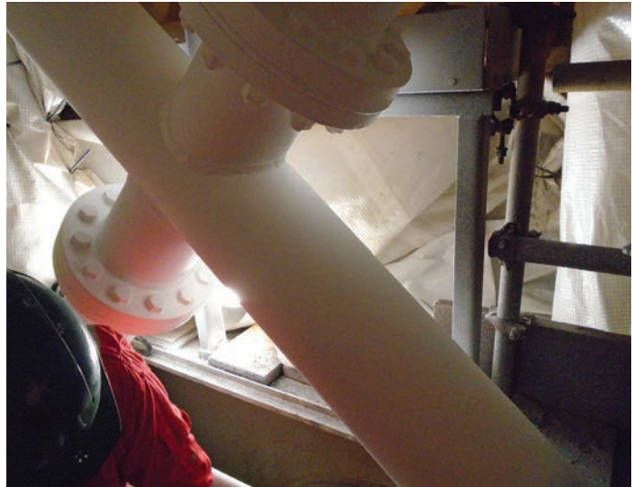
OGTC conducted successful trials using EonCoat on Total and Nexen platforms in the North Sea. Here we see the coating during the application process, and after completion.
