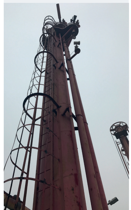
Fire Water Tower – before close-up
