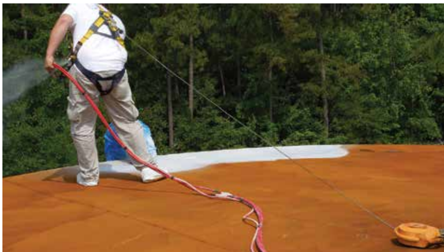
An alloy layer is formed making it impossible for corrosion promoters like oxygen and humidity to get behind the coating the way they can with ordinary paints.
