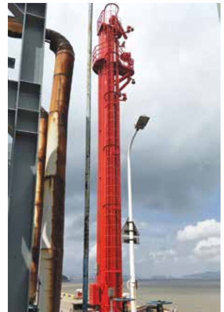
When the Xinao Group sought long term, external, corrosion protection for two firefighting water tanks, the company turned to EonCoat.
