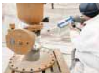
The spray-applied inorganic primer, EonCoat®, is a Chemically Bonded Phosphate Ceramic (CBPC), a new category of coatings designed to stop corrosion.
