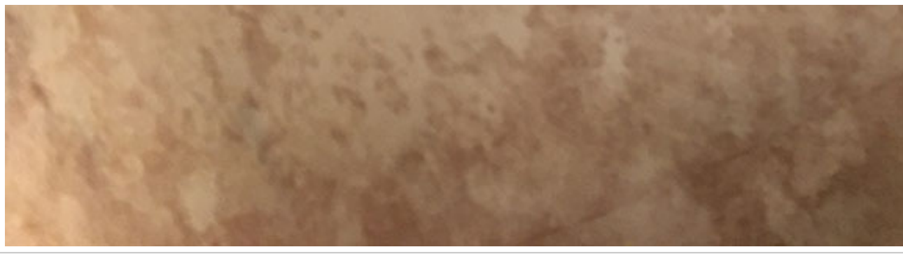
EonCoat - DFW Tank before.
