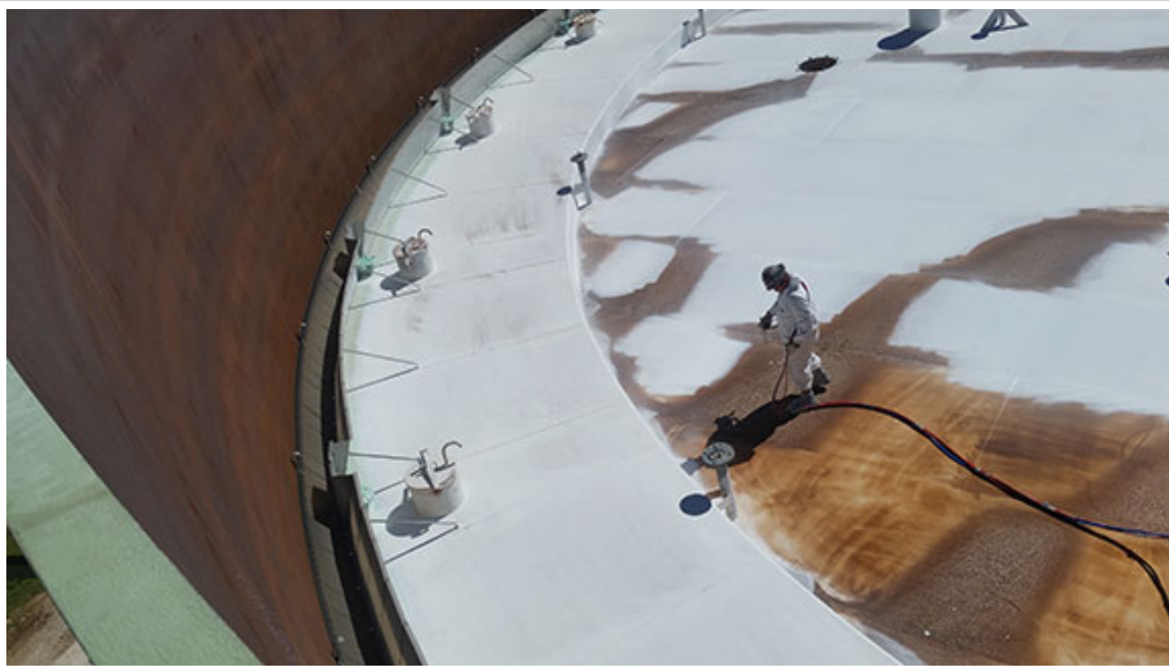
EonCoat application on tank
