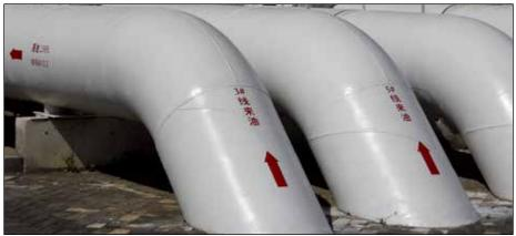
plural spray system like those commonly used to apply polyurethane foam or polyurea coatings. Since CBPC coatings are inorganic and non-toxic, there are no VOCs, no HAPs and no odor. This means the water soluable, non-flammable coatings can be applied safely even in confined spaces.
