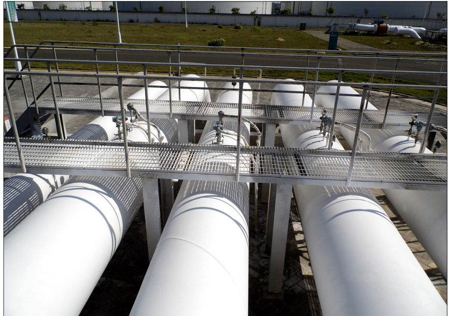
Figure 1 Chemically bonded phosphate ceramics provide an anti-corrosion coating for carbon steel pipes
