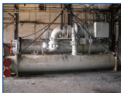
Two 800 Ton Mcquay Chillers, Water Cooled - Item: 40196 & 40197
