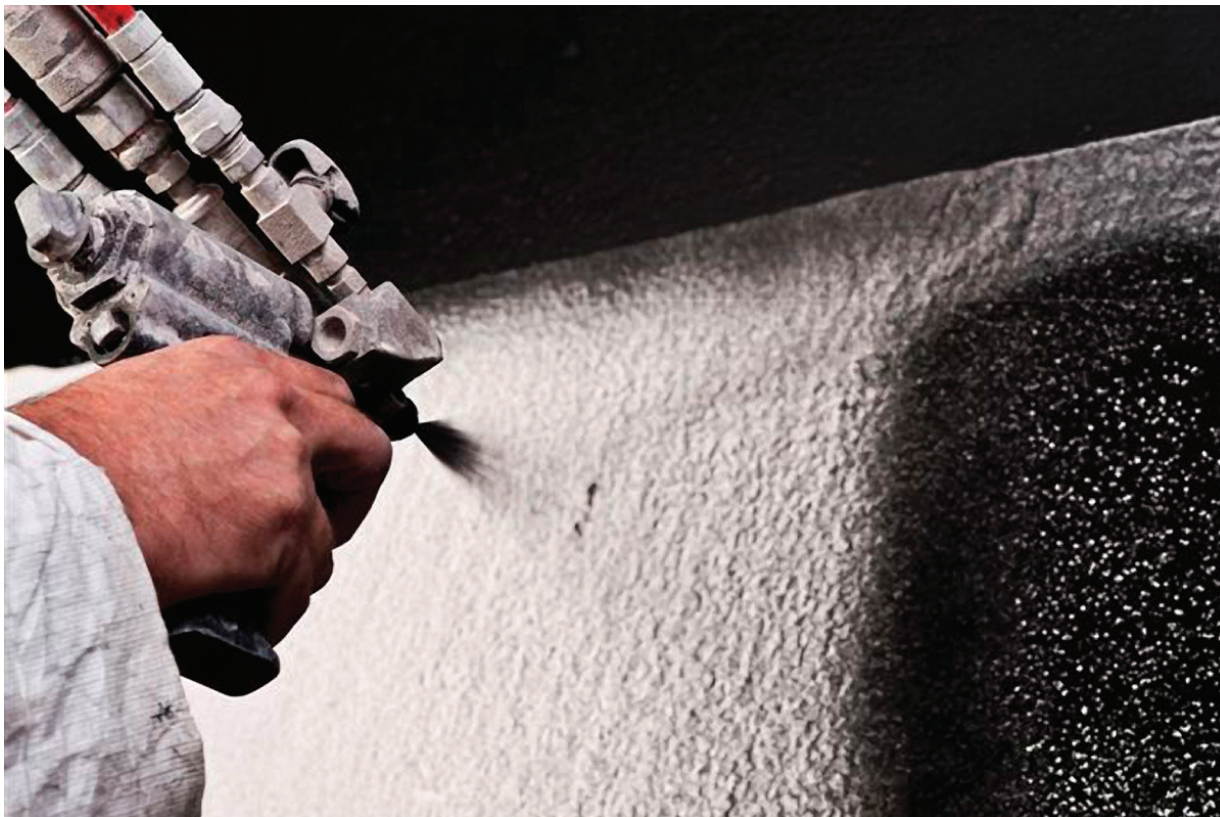
The ceramic coating for corrosion control consists of two non-hazardous ingredients that don't interact until applied by a plural-component spray gun.
